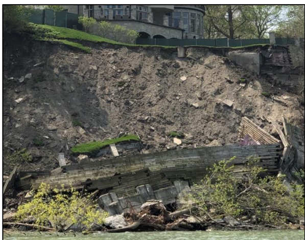
2020 Landslide – Failed Retaining Walls
