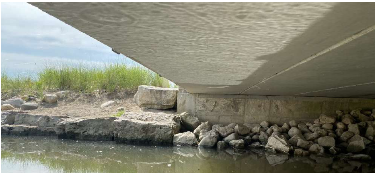
Photo 8 – Bridge Adjacent to Boardwalk
