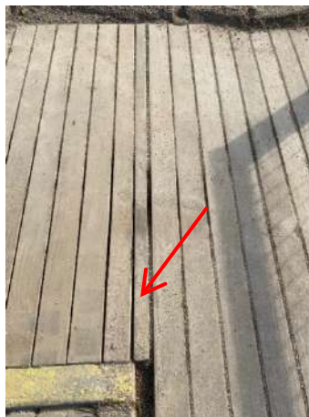
Photo 7 – Filler Board Installed in Boardwalk Gap
