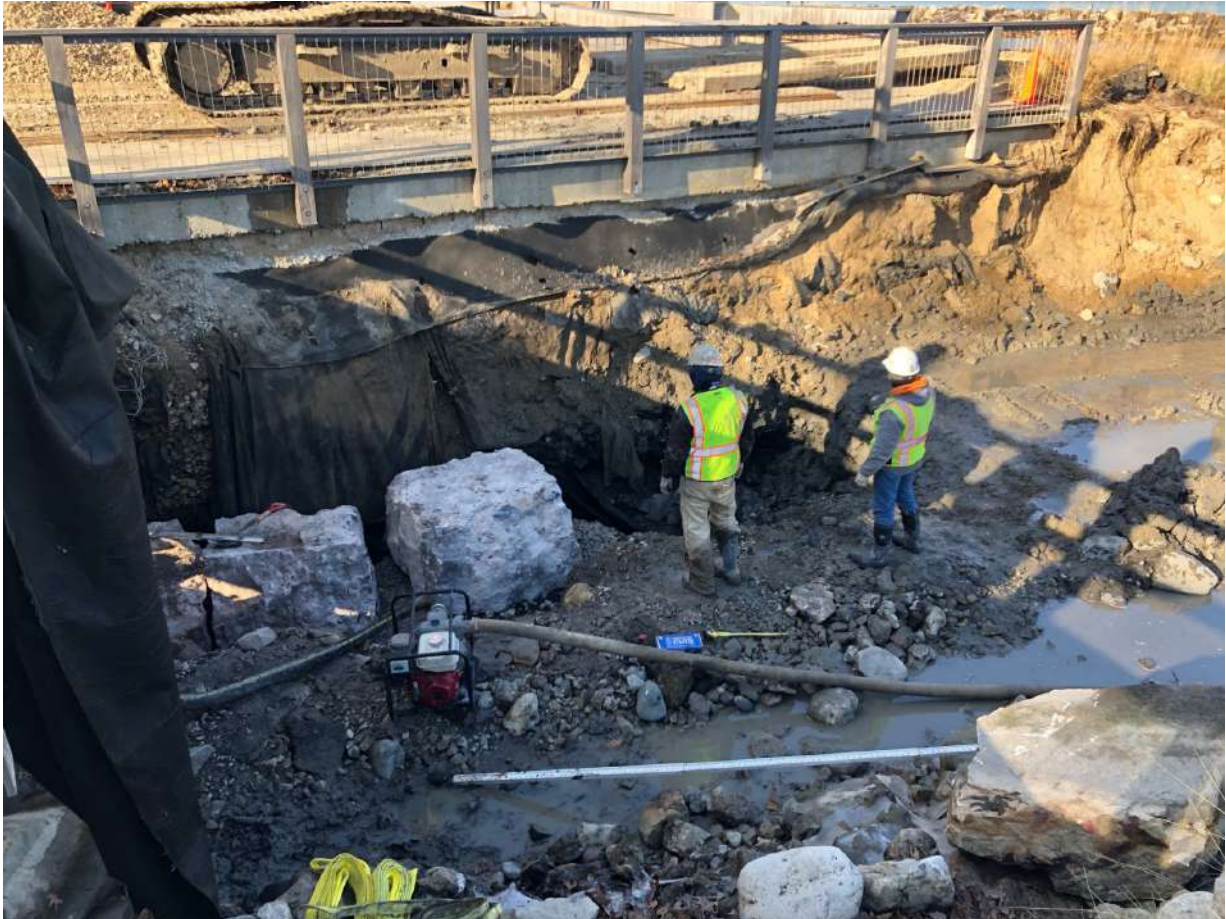
Photo 2 – Construction Photo of USACE Ravine Repair October 20, 2018
