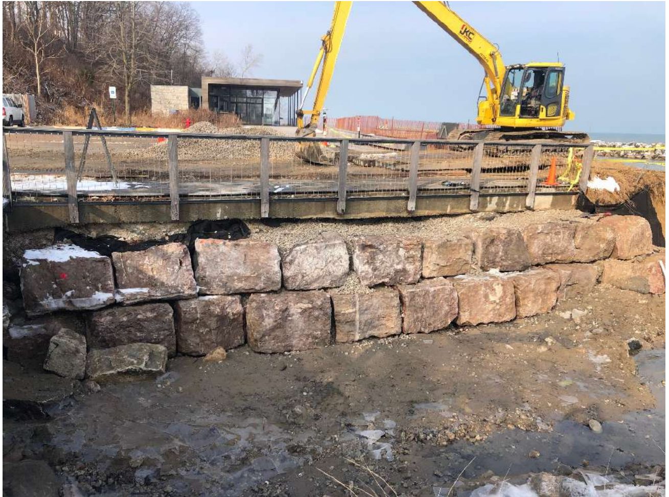
Photo 4 – Construction Photo USACE Ravine Repair, October 30, 2018
