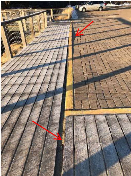
Photos 5 (left) and 6 (right) – Boardwalk Gap Due to Settling Toward Ravine, March 12, 2019
