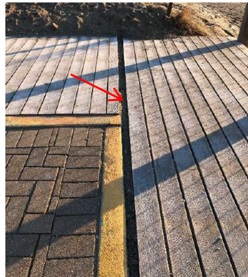
Photos 5 (left) and 6 (right) – Boardwalk Gap Due to Settling Toward Ravine, March 12, 2019
