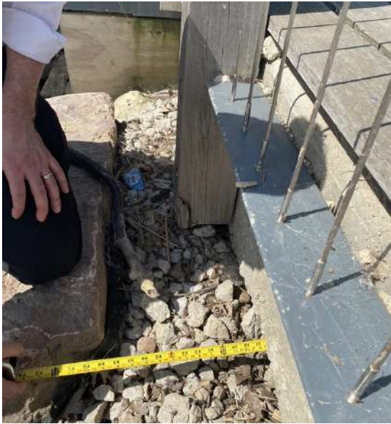
Photos 9 (left) and 10 (right): Open Space Between Aggregate and Concrete Slab
