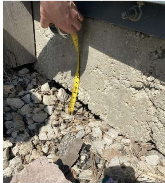
Photos 9 (left) and 10 (right): Open Space Between Aggregate and Concrete Slab
