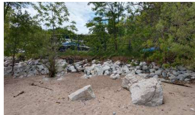
Figure 4.2 Remnant revetement stones on the north beach
