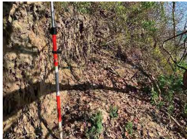
Figure 2.11 Slope failure at top of bluff on north end of Section C.
