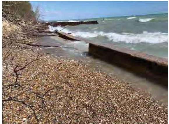
Picture 14: Washout occurring behind the seawall on the south of Section B.
