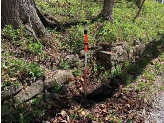
Figure 2.34 Drainage inlet found along Millard Park path.
