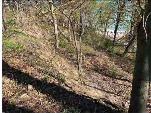
Picture 2: Slope Failure.
